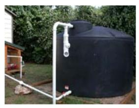
The District collects water off a 640 sq. ft section of roof. The water is gravity-fed into a 1550-gallon black polyethylene tank, which becomes nearly full after a 4 in. rain. We chose this lightweight, dark-colored tank in order to prevent the growth of algae. It measures approximately 7'-6" in diameter by just under 6'-0" high.
