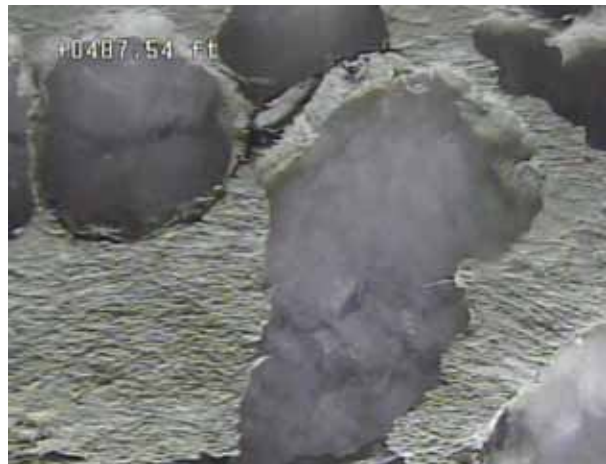
Figure 4. Photograph of a side view of a borehole showing evaporite (gypsum) nodules developed in the Upper Glen Rose. The photograph was taken at a depth of 150 m (490 ft) in the Hays MP well (Figure 1).
