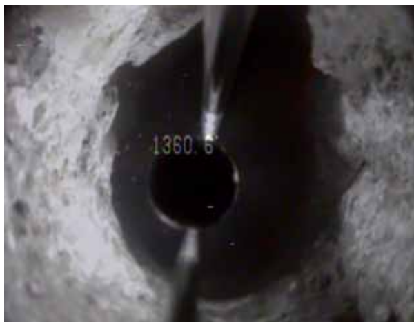
Figure 8. Photograph of a solution-enlarged fracture and void within the Cow Creek Limestone in a borehole at a depth of 400 m (1,360 ft).
