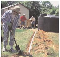
Mary Helen Quinn, Master Naturalist, helps dig the ditch for the PVC piping. Due to drainage issues, the tank needed to be located away from the building and downspout.
