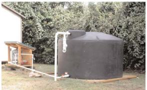
The District collects water off a 640-sq. ft section of roof. The water is gravity-fed into a 1550-gallon black polyethylene tank, which becomes nearly full after a 4 in. rain. We chose this lightweight, dark-colored tank in order to prevent the growth of algae. It measures approximately 7<sup>-6</sup>" in diameter by just under 6<sup>-0</sup>" high.
