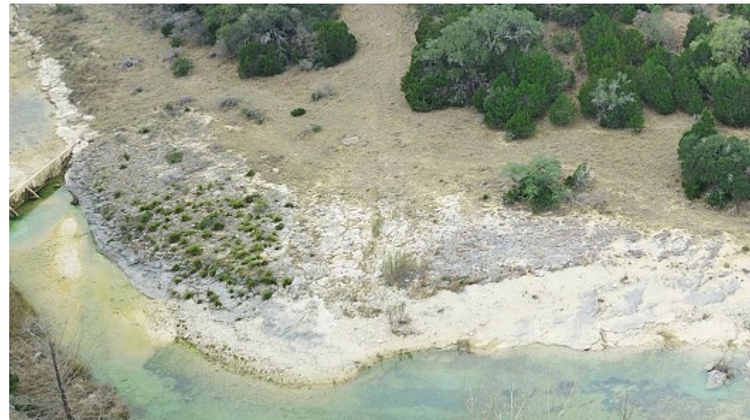
Existing KM pipeline in Blanco County
