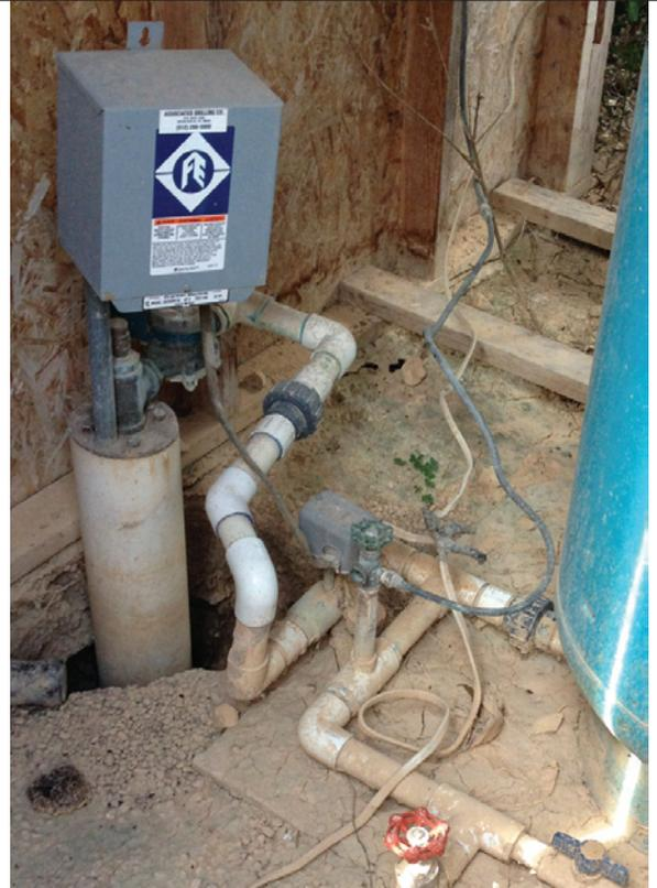
*A deteriorated annular seal around a well casing.*
