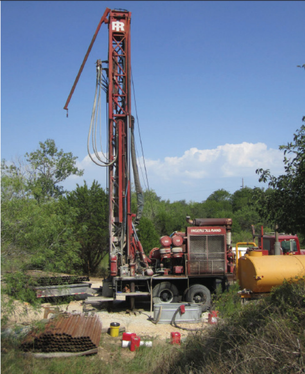
Drilling rig drilling a well in 2011.
