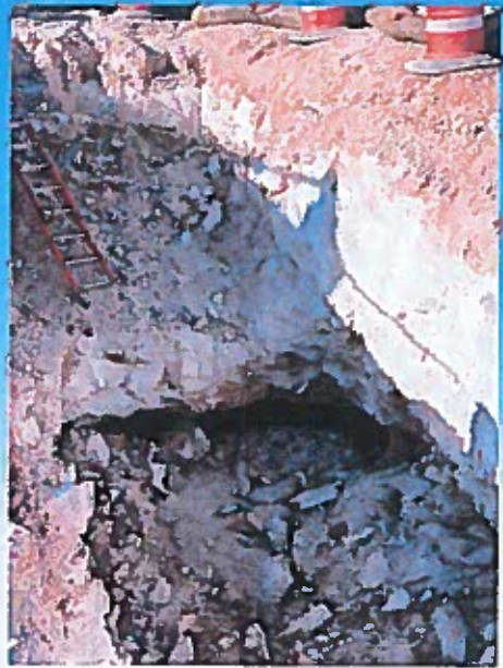
Void in the bottom of trench for water pipeline installation
