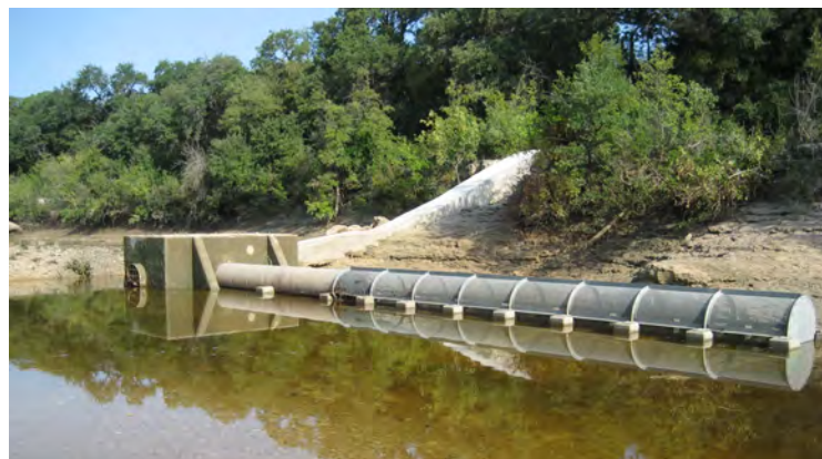
Figure 5. Antioch Cave recharge enhancement structure. Photo taken September 2010.
